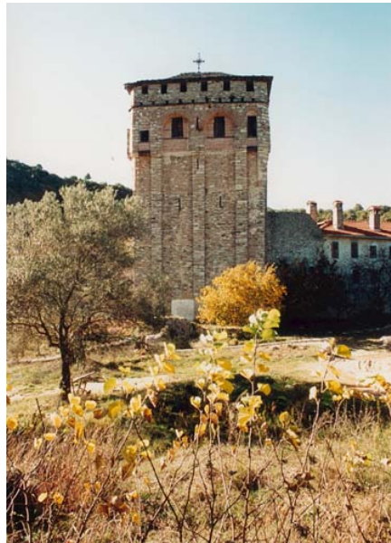
The tower of Chilandar Monastery - Serb monastery on Mount Athos
